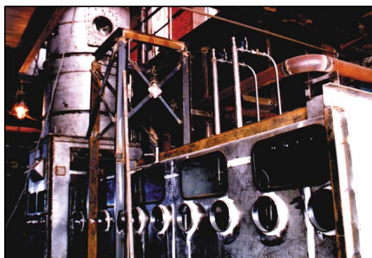
Industrial plant for destruction of mixed organic wastes containing natural uranium with a capacity of 50 t/y (Novosibirsk Chemical Concentrates Plant Ltd.)
